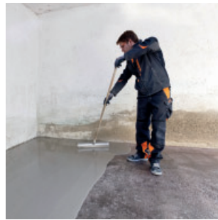
Distribution of leveling compound
