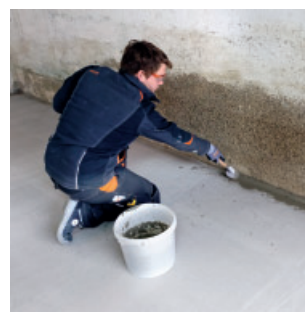
Installation of concave molding
