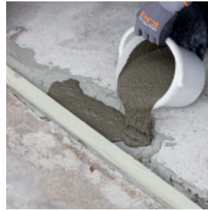
A screed rail is grouted using a flowable mortar
