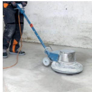
Grinding the floor
