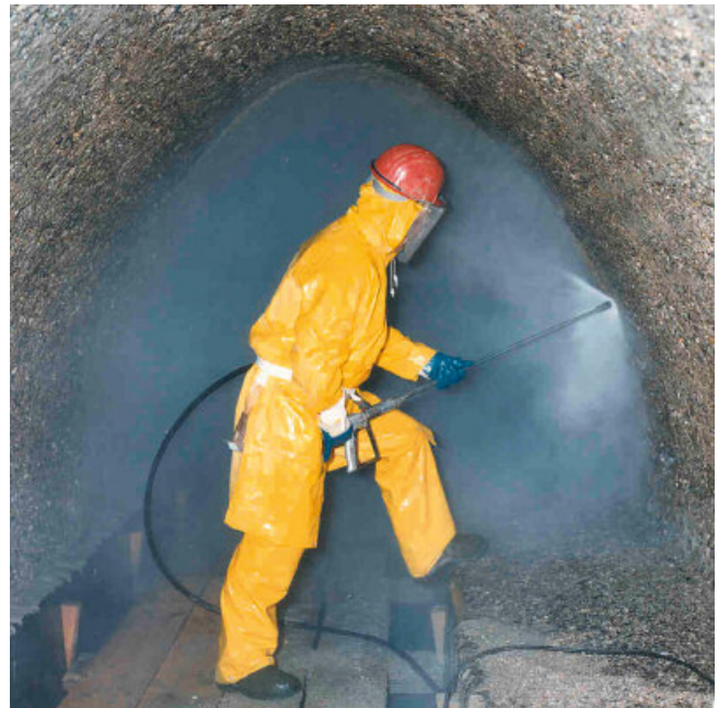
The largest grains in the aggregate should be exposed but should still be firmly anchored in the concrete matrix.
