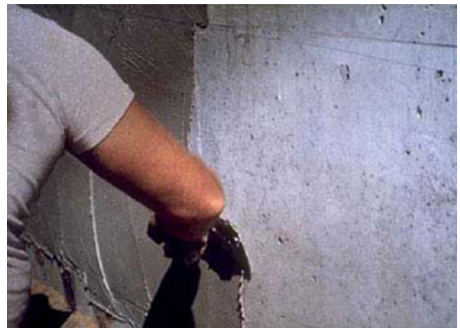
Interior waterproofing using PCI Barraseal®
