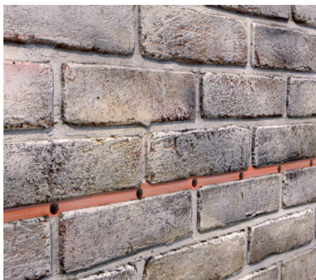
3. PCI Barra® Creme horizontal barrier following film formation.
