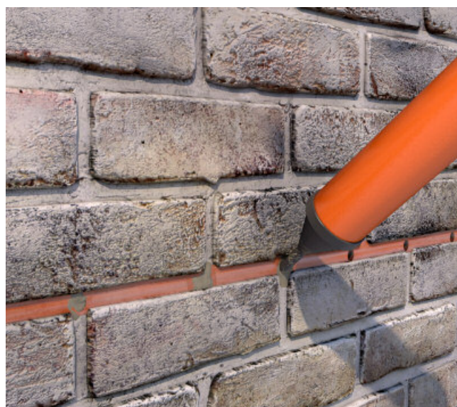
4. Sealing holes with PCI Barra® Inject cementitious suspension.
