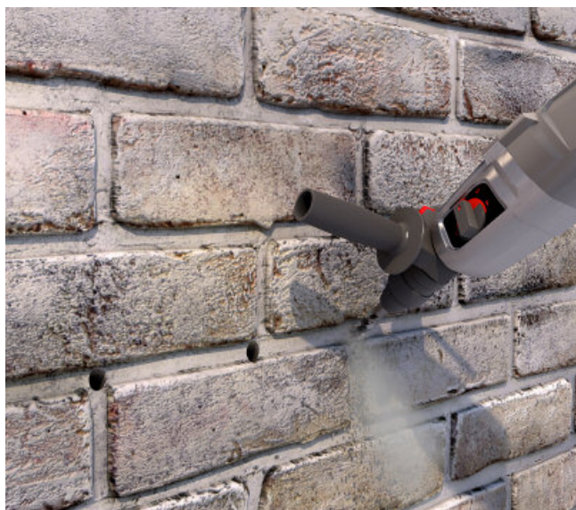
1. Drill holes and blow out any dust.
