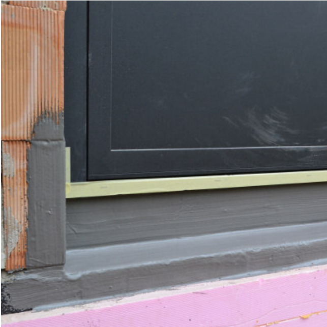
Joint with full-length window using PCI Barraseal® Turbo
