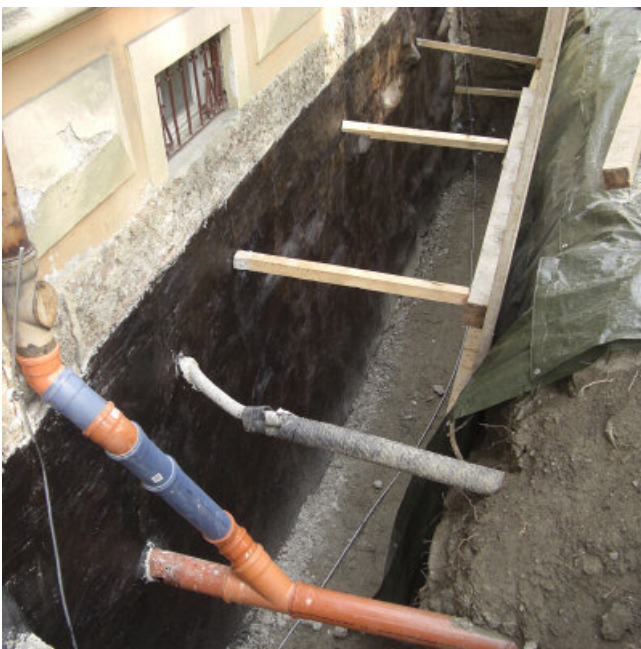
PCI Barraseal® Turbo reactive waterproofing on old waterproofing layers
