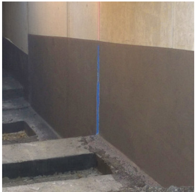
PCI Barraseal® Turbo for waterproofing wall surfaces
