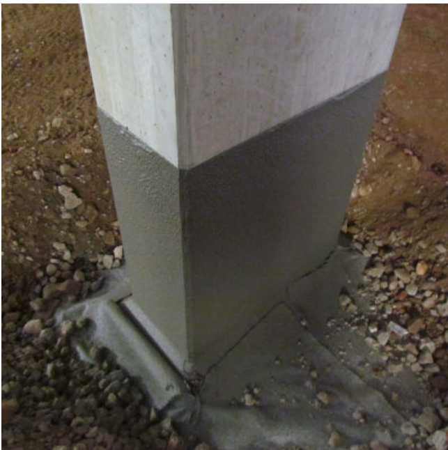
Protection of concrete surfaces in accordance with OS 5b with PCI Barraseal® Turbo
