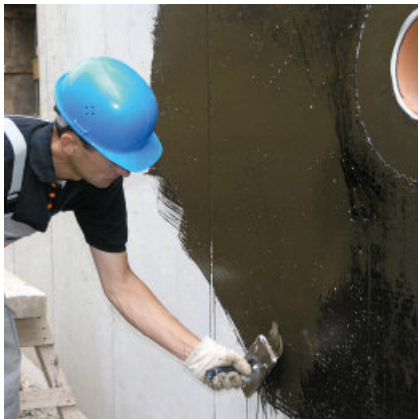
Priming in the summer: PCI BT 26, priming in the winter: PCI BT 28 special primer
