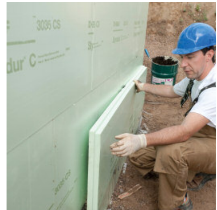
Bonding of insulation boards using PCI Pecimor® DK
