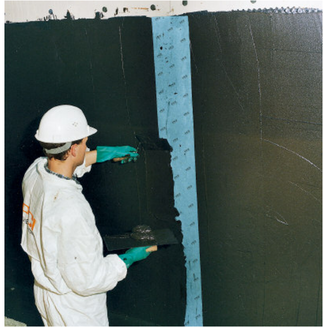
Insertion of Pectitape® 250 waterproofing tape over a joint
