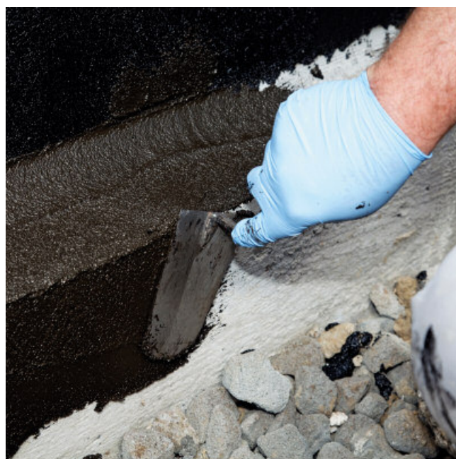
PCI Pecimor® waterproofing must be continued to a depth of at least 15 cm on the foundation slab
