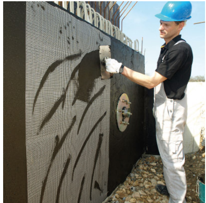
Application of reinforcing fabric to fresh PCI Pecimor® 2K thick bituminous coating
